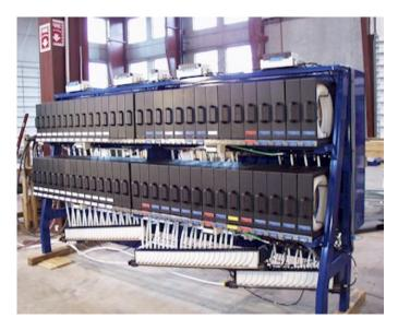
Figure 3. A 60 Slot CFAS rack with PLC control
