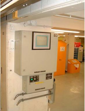
Figure 4, Hydraulic enclosure (top) Electrical enclosure (bottom) typ each arm. 4 locations include operator touch screen.
