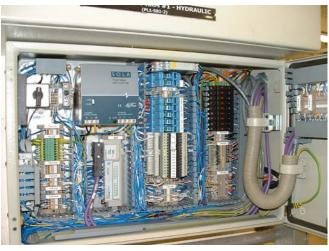
Figure 7, Electrical controls typical each arm.
