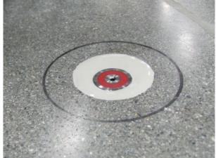
Figure 7 – Floor Resynchronization Target
