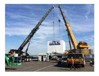
Figure 12 crane layout for the machine lift at the Boeing Renton site.
