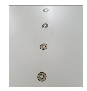
Figure 6. Blind fasteners installed and shaved flush with the OML
