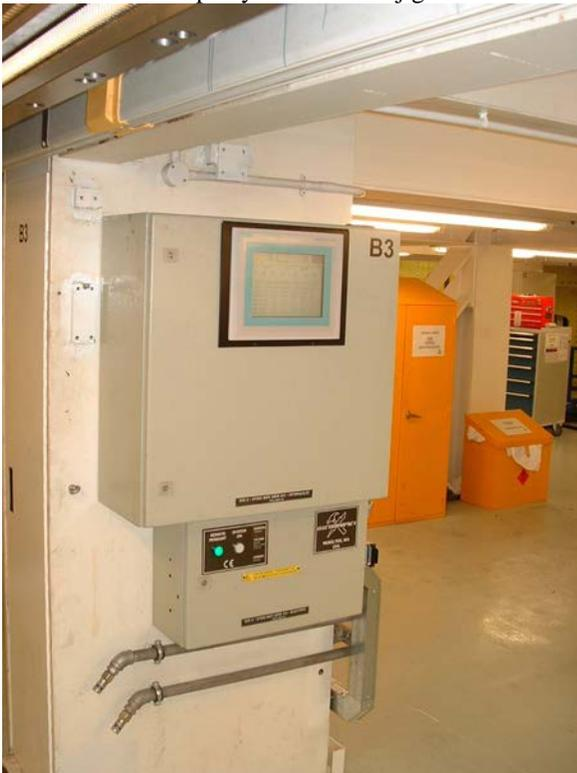
Figure 4, Hydraulic enclosure (top) Electrical enclosure (bottom) typ each arm. 4 locations include operator touch screen.
