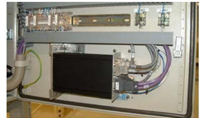
radiomatic wireless pendant and hydraulic pump as it removed the requirement of passing information between separate controllers. The controller is a Siemens CPU315-2DP with integrated Profibus. The HNC's and any other I/O connect to the PLC via this single Profibus. The total length of the Profibus network is 400M and it runs at 500kHz.
