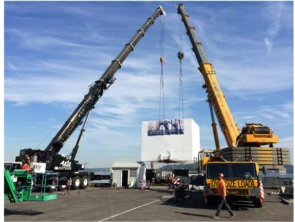
Figure 12 crane layout for the machine lift at the Boeing Renton site.
